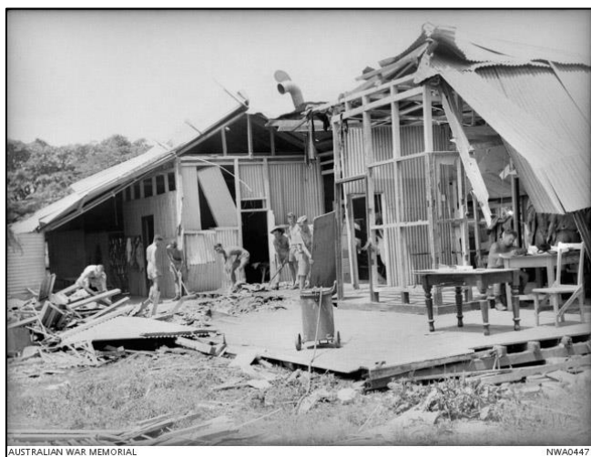
Australian servicemen in Darwin repairing a bombed building after the second air raid by Japanese warplanes on 19 February 1942. These were possibly huts at the RAAF base. AWM NWA0447
