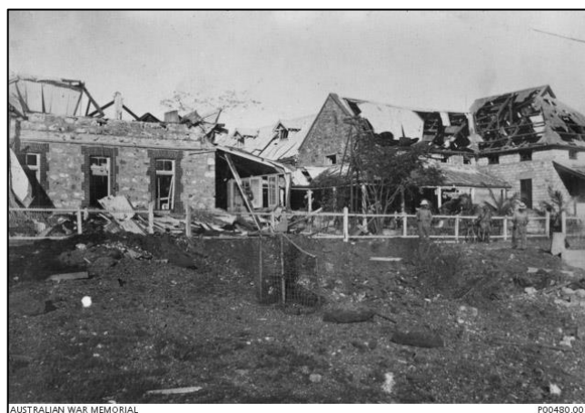
People survey the bombed Post Office and postmaster's residence where 9 people died after the first Japanese air raid on Darwin on 19 February 1942. AWM P00480.001
